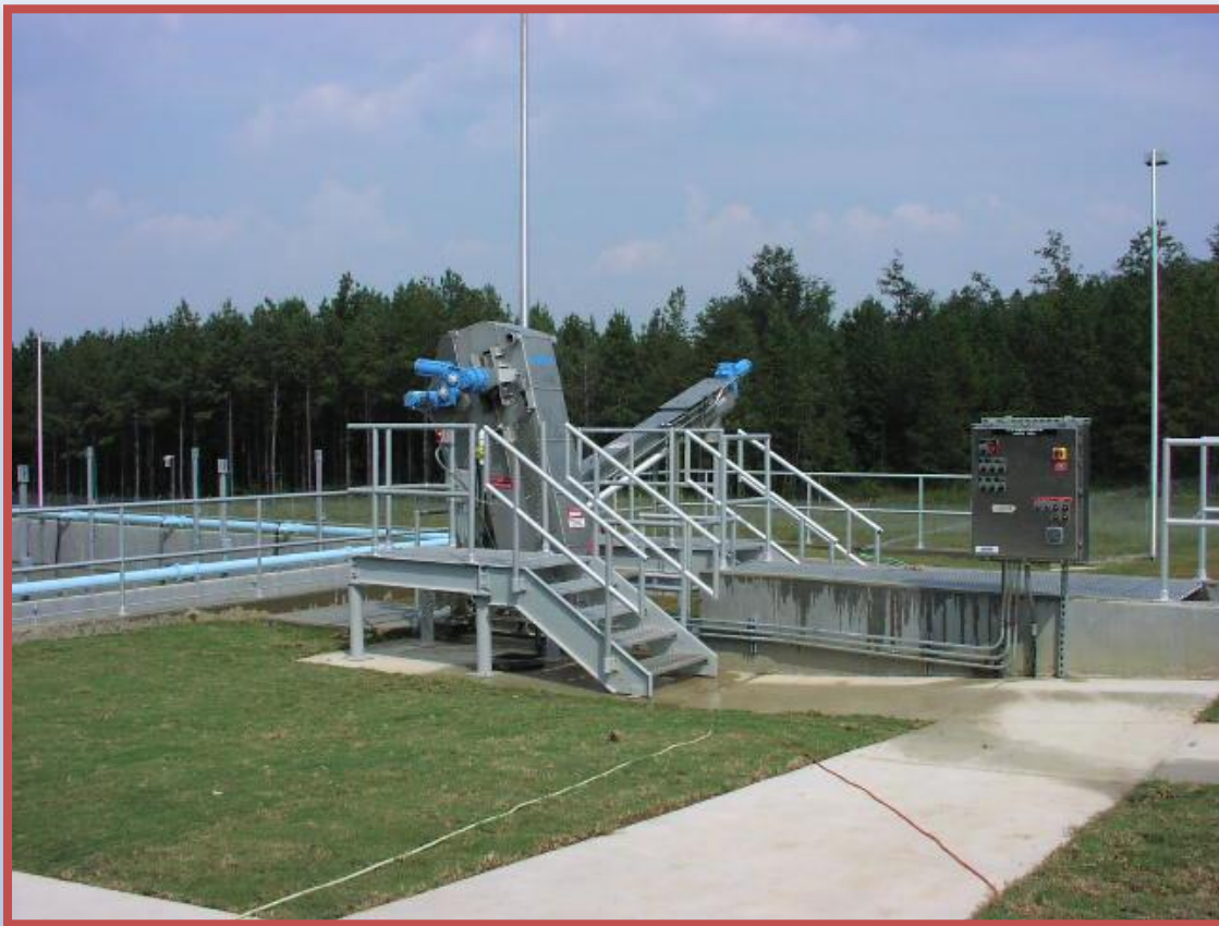
Wastewater Treatment Facility
